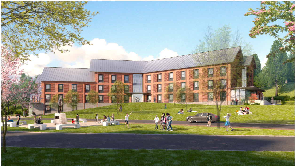
Dormitory and Wellness Center to be completed in Spring 2024
